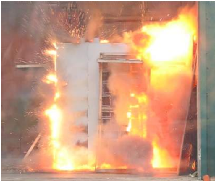
Fig #1 - 65kA Bus Compartment Arc
