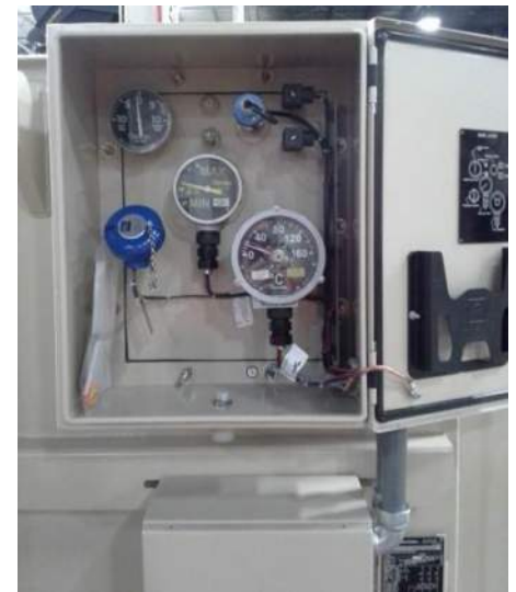
Load-break switch handle
